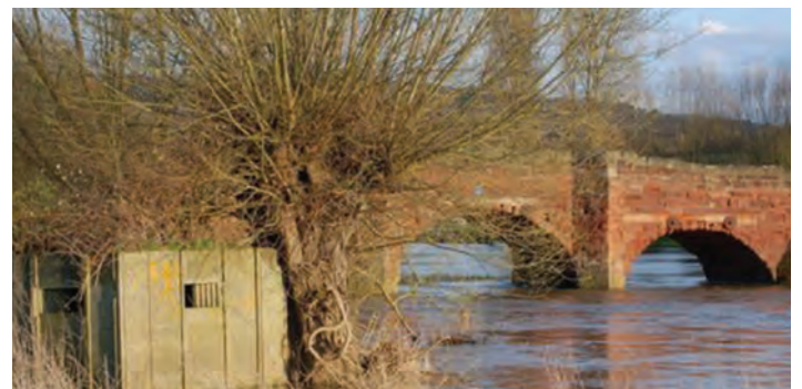
Pillbox, Eckington Bridge
